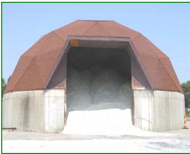
Deicing materials storage bunker
